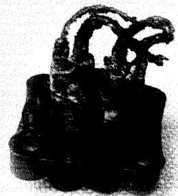
Photo showing acid attack on the compressor's terminal wires
