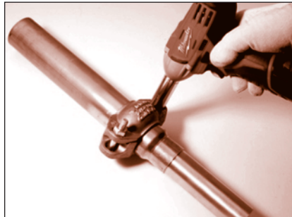
FIGURE 43: Tightening the clamp
